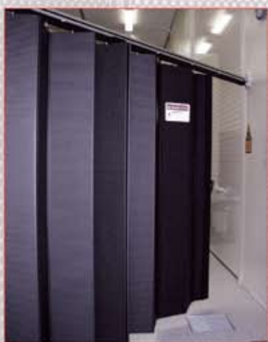
short curtain segment to shield entry
